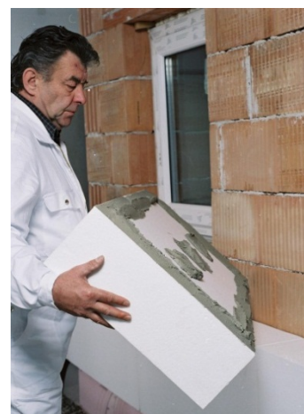
Photo: WDVS processing
