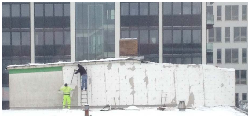
Photos: Deconstruction of an ETICS
