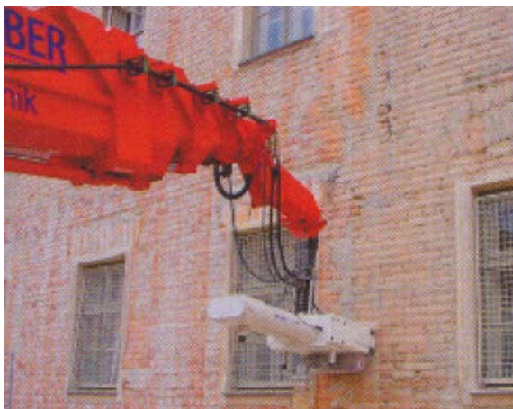
Photo: Milling cutter in operation
