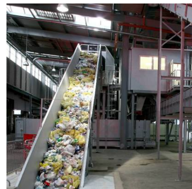
Photo: Waste sorting plant
