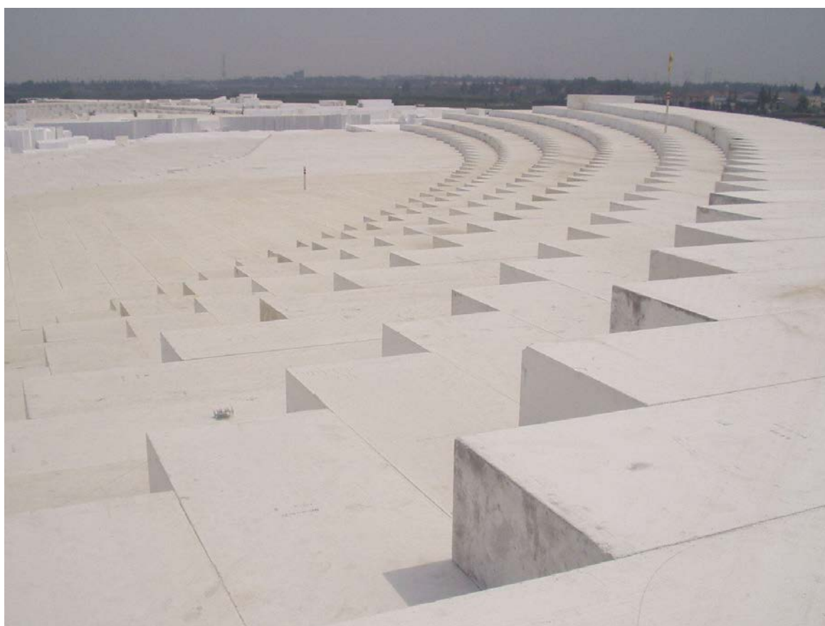
Photo: Grandstands for the Shanghai Formula 1 course under construction
