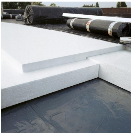
Photo: Pitched roof
