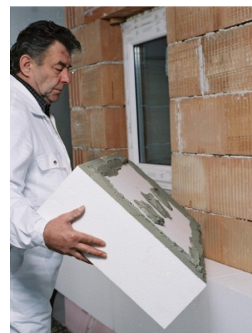
Photo: WDVS processing
