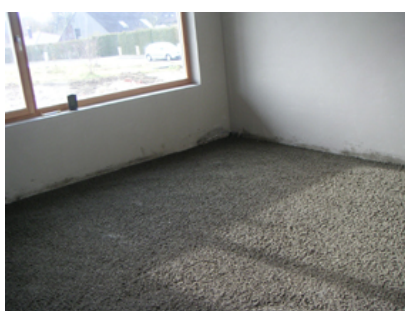
Photo: Bound EPS ballasting
